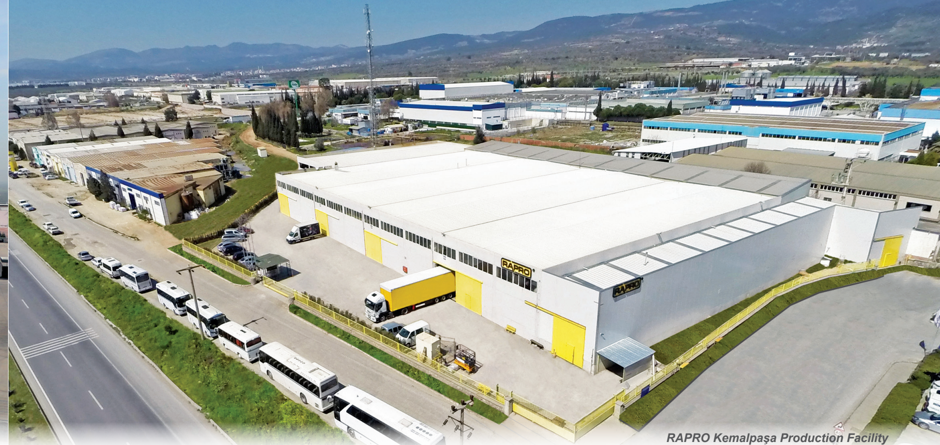
RAPRO Kemalpaşa Production Facility
